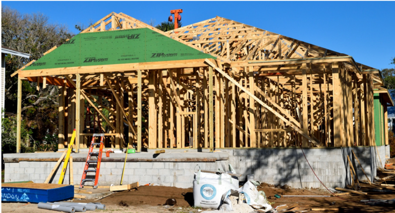
Figure 150 Framing a House upon a Solid Foundation
